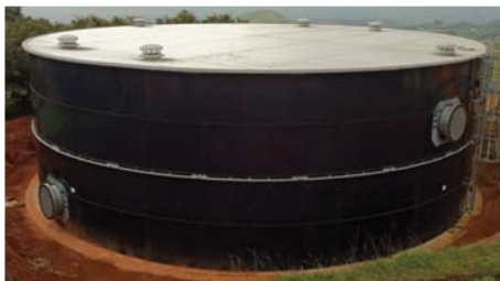
Trough Deck Roof
